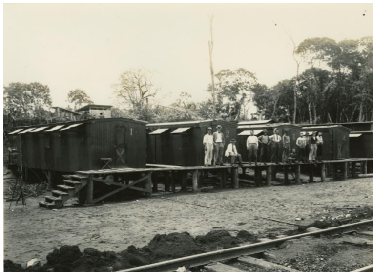
Figure 4-4. A construction camp for Railroad employees assembled out of old box car bodies then used as living quarters, 1910. Courtesy of the Panama Canal Museum Collection, University of Florida.
